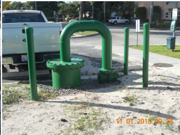
Completed Disposal Well #1
