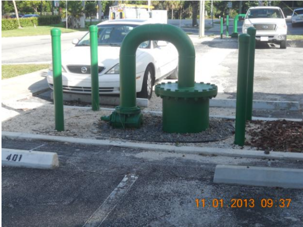
Completed Disposal Well #2
