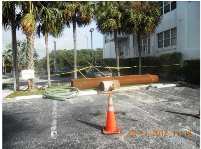
24 " dia. X 20' long steel pipe for well casing.
