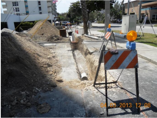
Trench work for new 10" dia. connector pipe.
