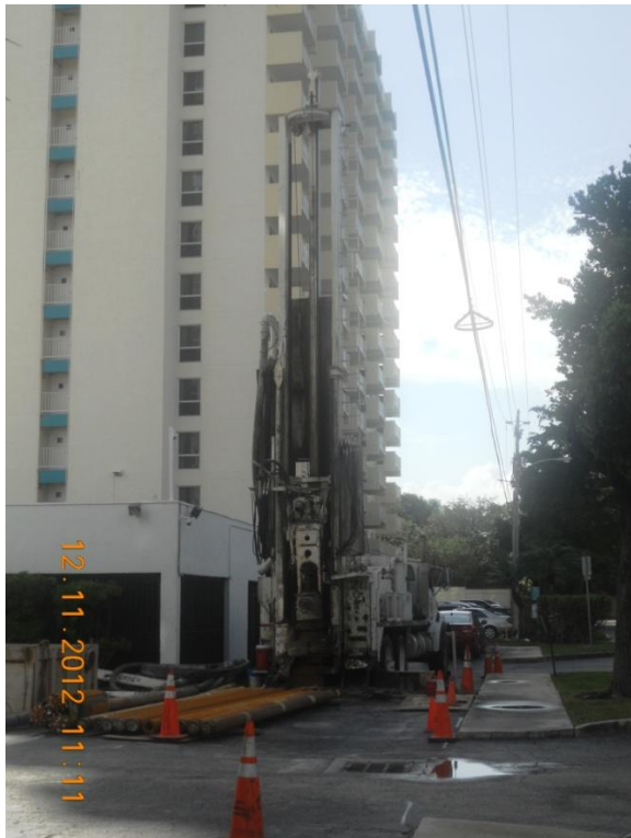
Drill Rig set up on SW corner of property
