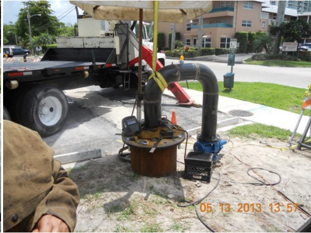
Trench backfilled and connected to supply wells.
